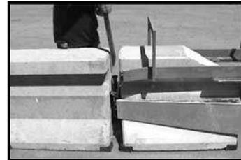
1.13 Tap the top of the pin with a pry bar to ensure the pin is fully installed.
