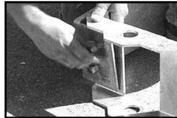
1.6 Attach the Nylock nuts on the ends of the bolts. Make sure to install the nuts on the outside of the strap as shown and hand tighten.
