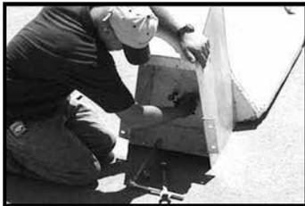
1.6 Tighten the nuts on the Anchor Bolts so that the adapter is tight against the PCB.
