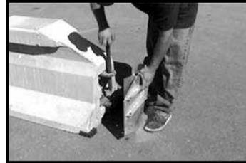
1.1 Remove the pin from the sloped end of the QMB Attachment Barrier
