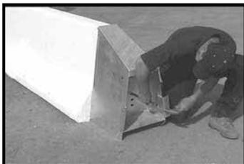
1.8 **OPTION:** In the event that the Taper Adapter is installed on a permanent concrete wall, mounting bolts must be installed. Place the Taper Adapter against the wall in its proper position.
