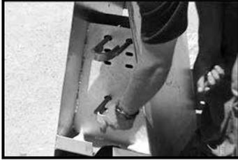
1.1 Insert the Anchor Bolts through the holes in the adapter. There are two sets of holes in the adapter; use the holes on the top of each set.
