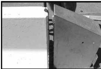
1.4 Align the Anchor bolt loops with the PCB loops so the pin can pass through all four of the loops. If there is interference due to the height of the Anchor Bolt loops.
