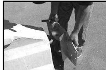
1.2 Fit the adapter plate over the hinge on the sloped end of the QMB Attachment Barrier.
