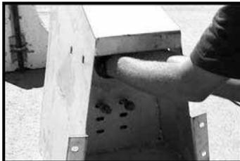
1.2 Install the nuts with washers on the end of the anchor bolts that are now on the inside of the transition.
