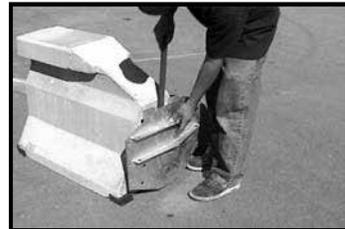
1.3 Secure the Hinge Plate Adapter to the Attachment Barrier by installing a QMB Hinge Pin.
