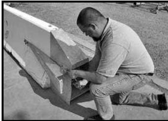
1.14 Tighten the Side Strap nuts and bolts on the steel transition housing.
