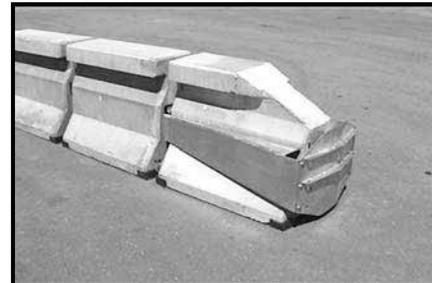
Fully installed QMB Attachment Barrier
