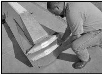
1.13 Remove the Hinge Plate Adapter that was loosely attached earlier.
