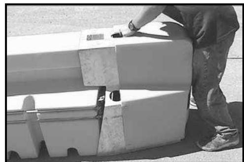
PCB Nose – Slide corners over the final element
