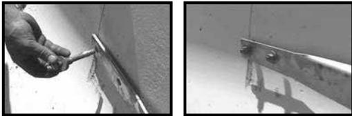
1.12 Now that the Strap Ends are at their final "level" position on the PCB, drill (4) 1/2" (12 mm) diameter holes, 3/4" (80 mm) deep in the side of the PCB. Install (4) 1/2" x 4 1/4" (12 mm x 108 mm) wedge anchor bolts. Place one 1/2" (12 mm) flat washer and nut on each anchor bolt. DO NOT TIGHTEN.
