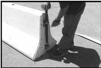
1.3 Remove the pin from the end of the PCB.
