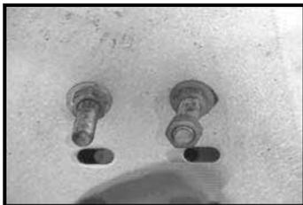
1.7 Tighten the four nuts on the Anchor Bolts to 15 ft-lbs (20 Nm). Then install a jam nut against the first nut with a torque of 40 ft-lbs. (55 Nm).
